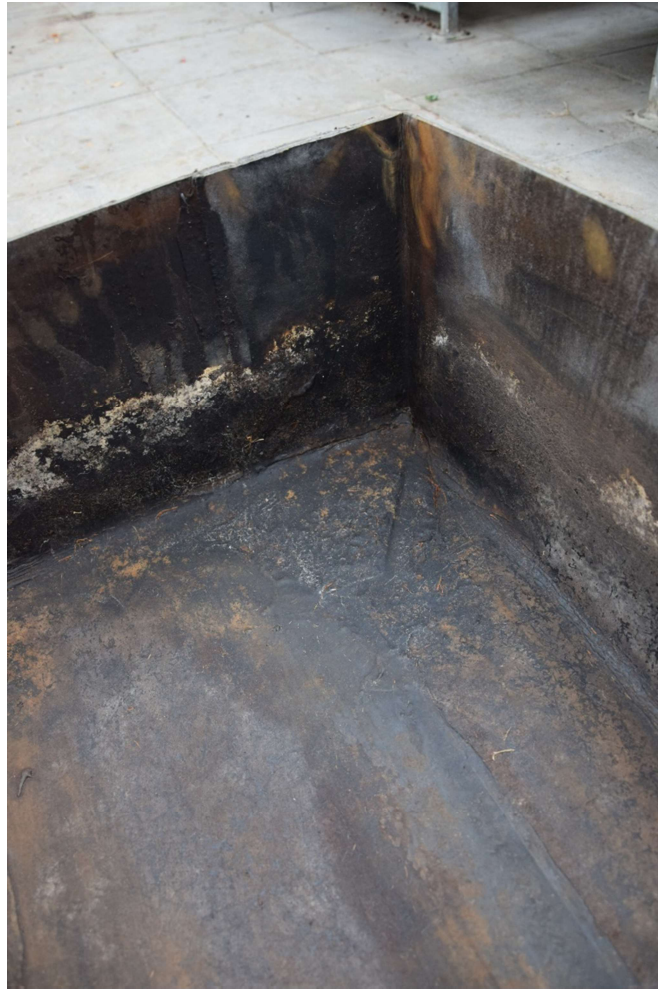
Fig. 3: Corner of the test specimen at the end of the test
