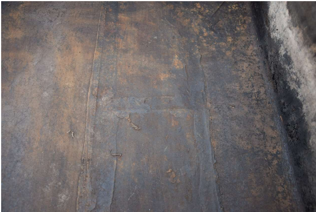
Fig. 2: T-joint at the end of the test
